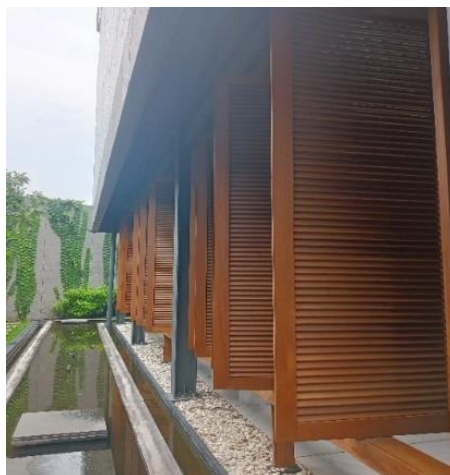
Wood and stone elements at the Saminah Sihyadi Mosque Source: Asran, 2025
