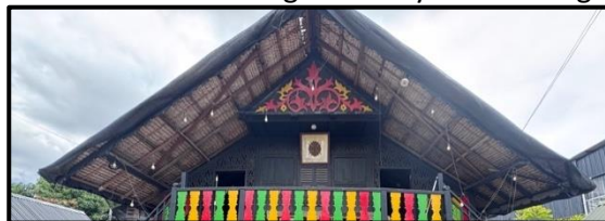
Figure 20. Roof of Rumoh Aceh Source: Author's Documentation, 2026
