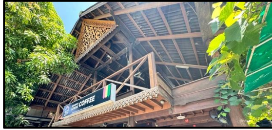
Figure 8. Roof of Rumoh Aceh Source: Author's Documentation, 2026
