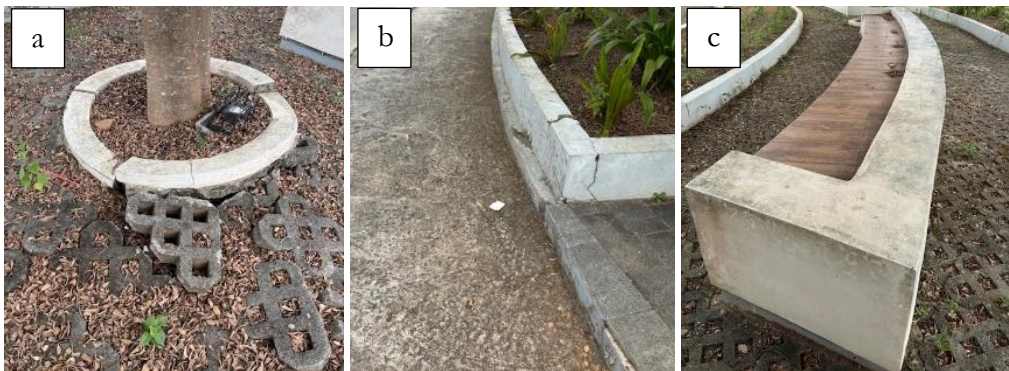
Figure 4. (a) Grassblock, (b) concrete curbs, (c) seating area
