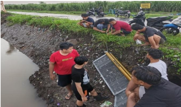
Gambar 4. Proses pemasangan river barrier
